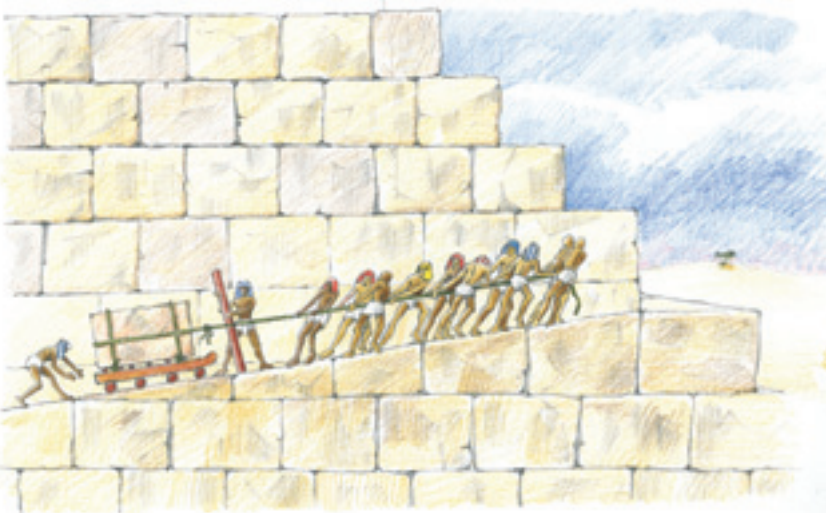
4,500 years ago, the Egyptians used simple machines to move three-ton stone blocks up the 150 m-tall Great Pyramid of Cheops. They constructed ramps of stone cubes or earth, and pulled and pushed the blocks up the ramps on wooden rollers.
