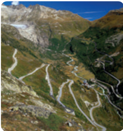
A switchback is a zigzagged inclined plane.
